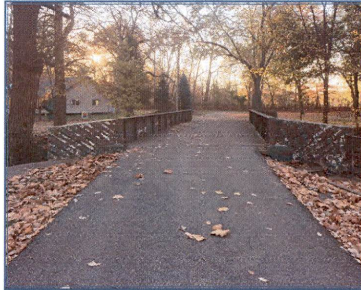
Bridge across Cedar Creek in Eckhart Park
